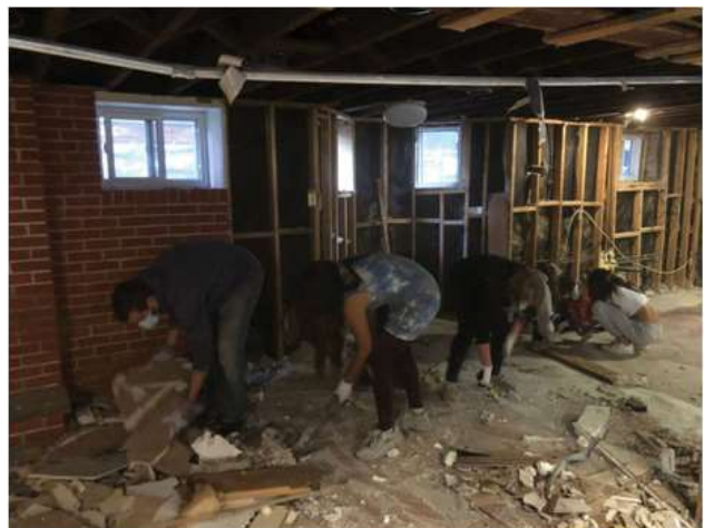
Adam House Renovation
